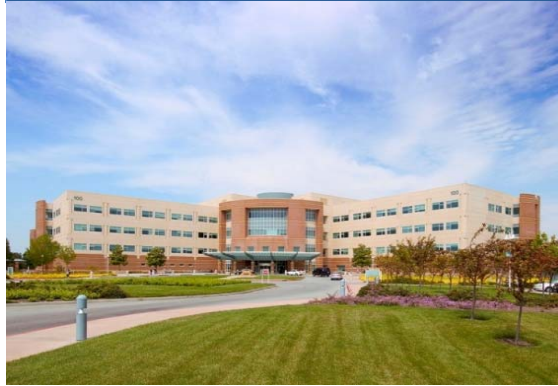
VA Palo Alto Health Care System Palo Alto, CA
